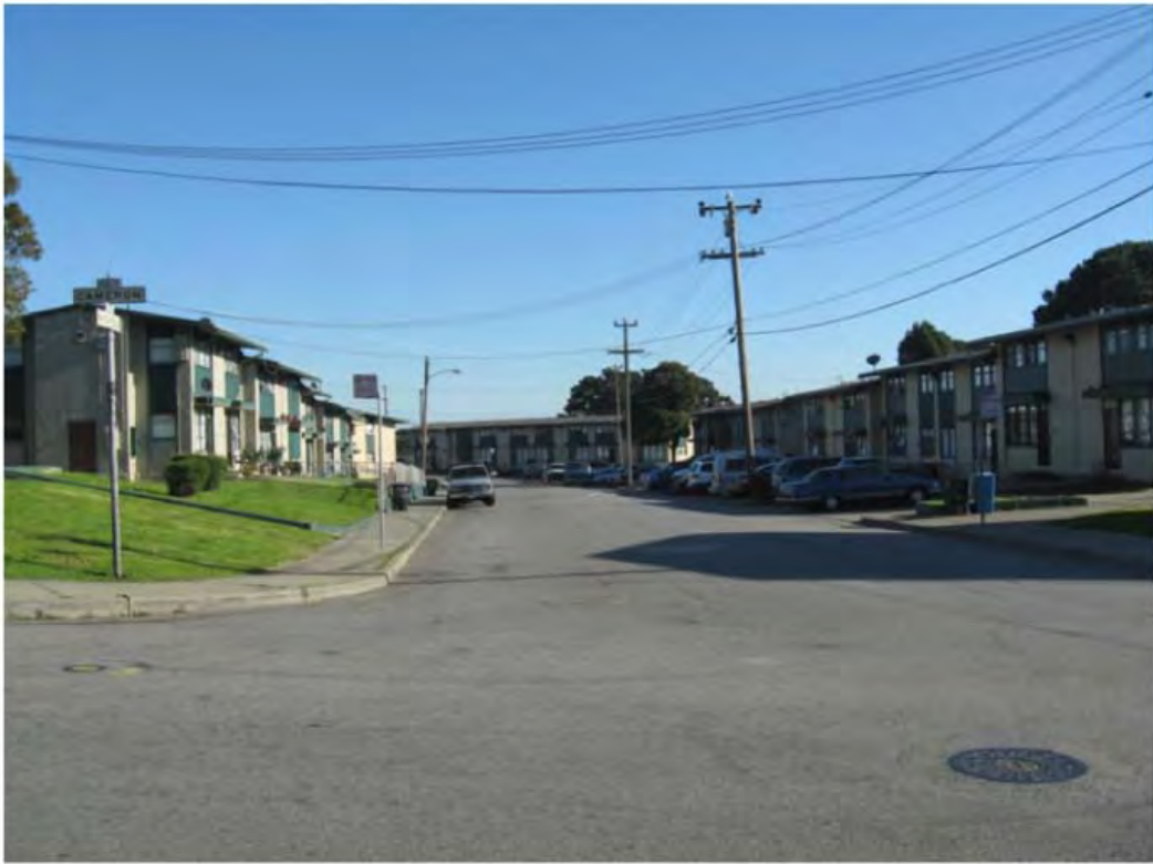
View (C) within Project Site, along Nichols Way, looking southeast from Cameron Way
