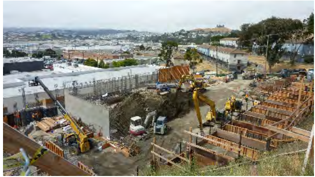
Potrero Block X construction as of June 2017
