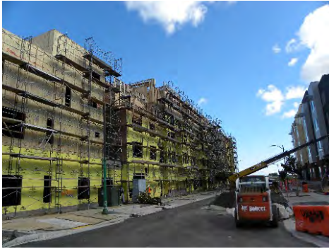
Alice Griffith Phase 3 under construction as of February 2017
