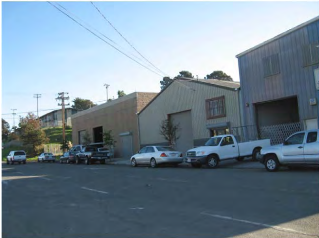
View (L) toward Project Site, looking southwest along Carroll Avenue (light industrial uses)
