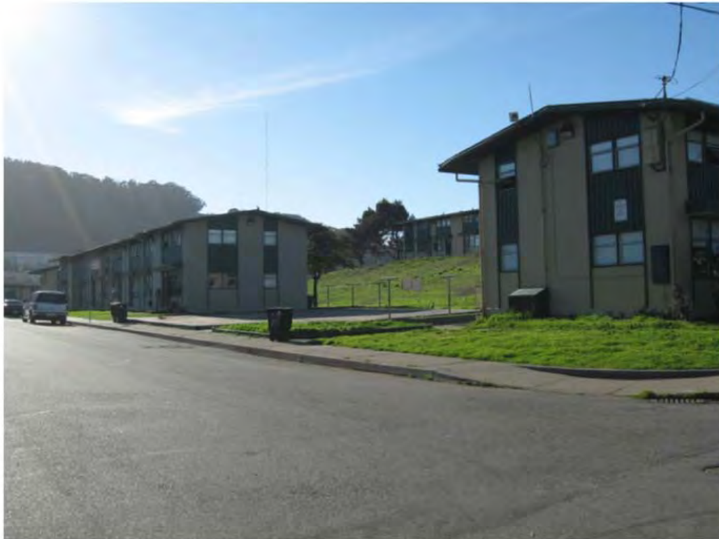
View (B) within Project Site, looking southeast from Cameron Way and Nichols Way Intersection
