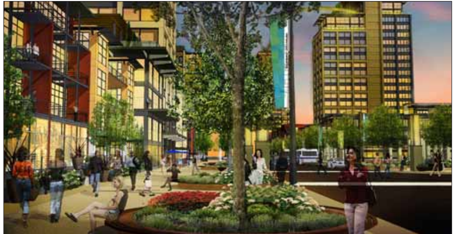
Candlestick North at the edge of the centrally located community park.
