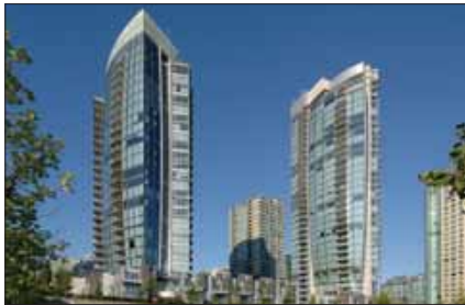
Precedent – Residential high-rise building.
