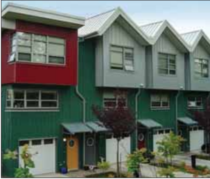
Precedent – Garage entrance off private driveway.
