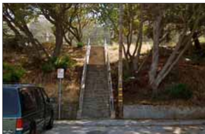
Gilroy Street Steps
