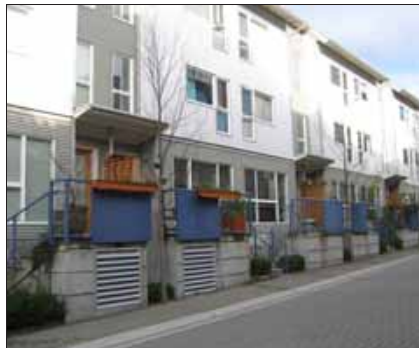
Precedent – Consistent palette of materials creates clear building identity.
