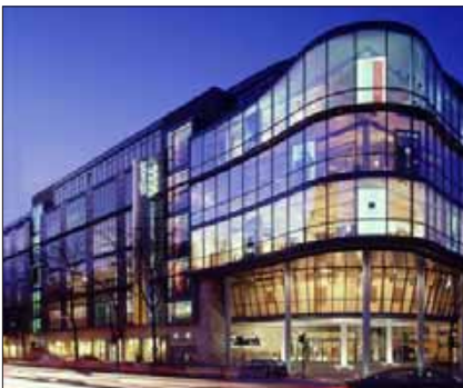
Precedent – Commercial at corner.
