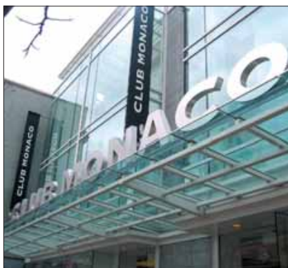
Precedent – Awning signage consistent with building architecture.
