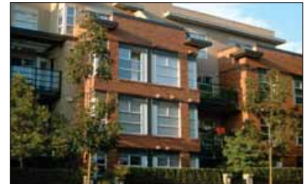
Precedent – Façade articulation.
