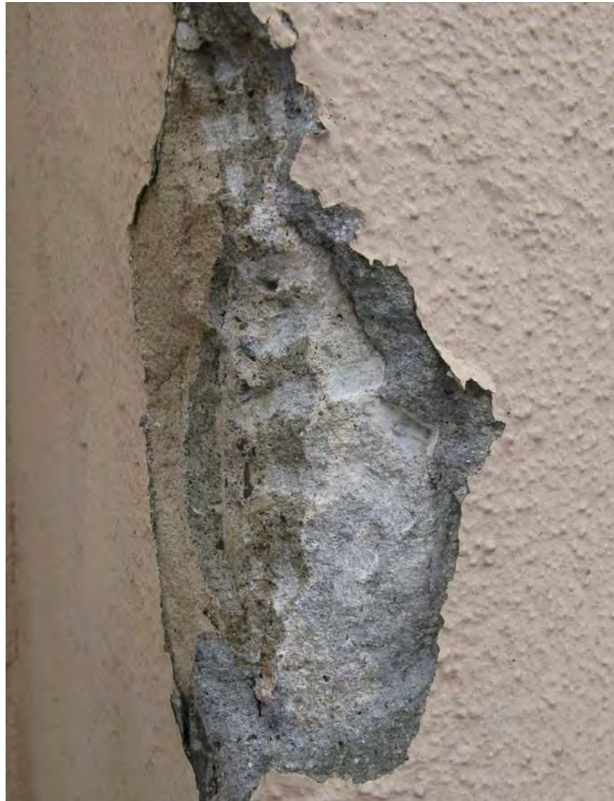
Sample 7: Concrete below layer of bedding mortar and cement stucco
