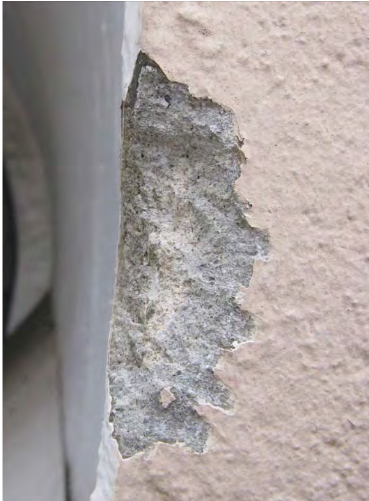
Sample 4: Cement stucco cut away to reveal white bedding mortar
