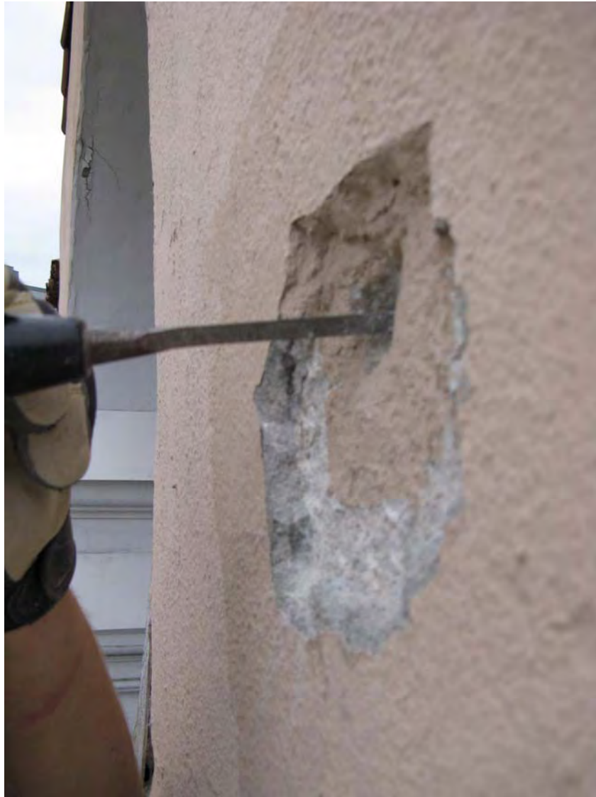
Sample 3: Cutting into concrete substrate
