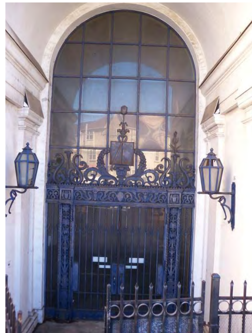
Figure 17. Main entrance to Woods Hall, 2012 Source: Christopher VerPlanck
