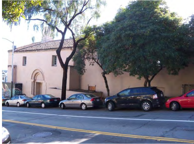
Figure 22. North façade of Woods Hall Annex, 2012 Source: Christopher VerPlanck
