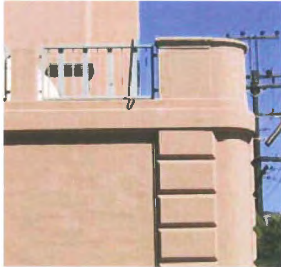
(E) Cement Plaster Example
