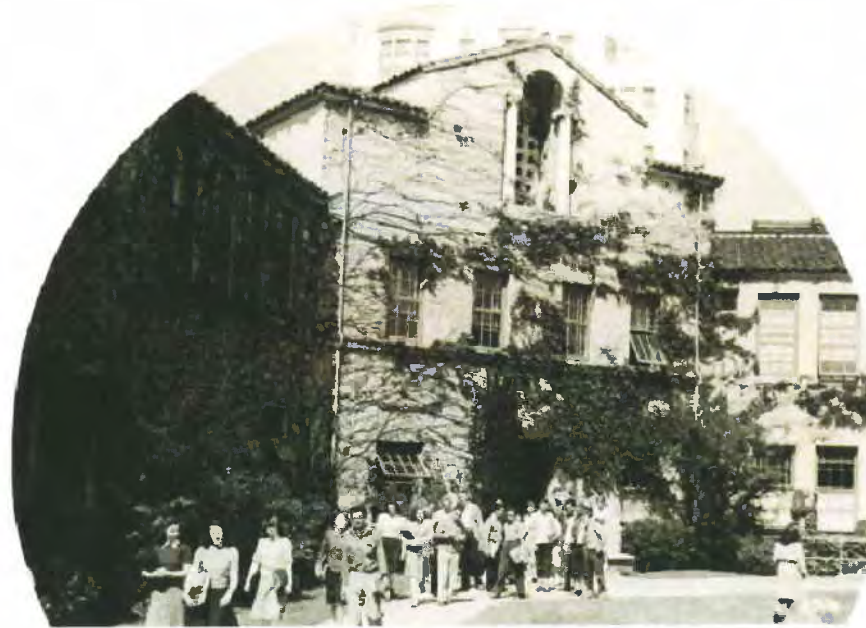
View of Woods Hall courtyard entry, 1941 (San Francisco Public Library)
