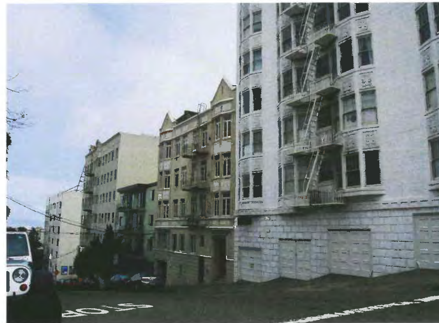
⑥ View from Buchanan and Hermann streets, looking southeast
