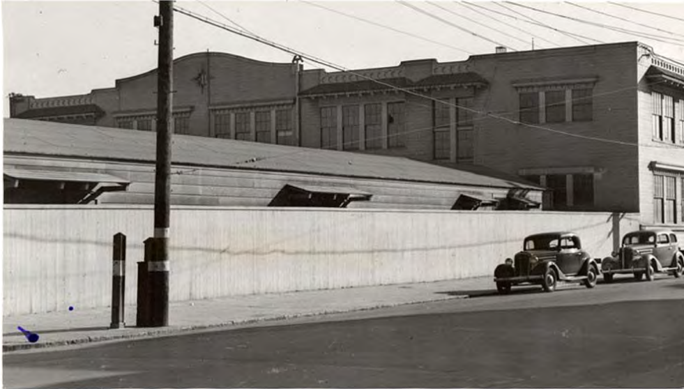
Figure 39. San Francisco State College, 1937; view along Buchanan Street showing the old Administration Building (background) and one of the “shacks” (foreground)
