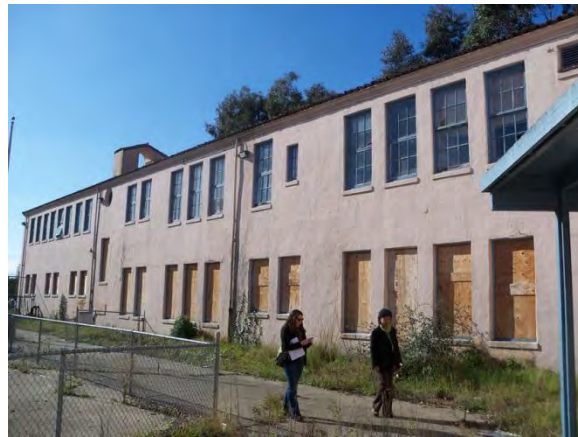
Figure 21. Courtyard (east) façade of Herbst Wing, 2012
