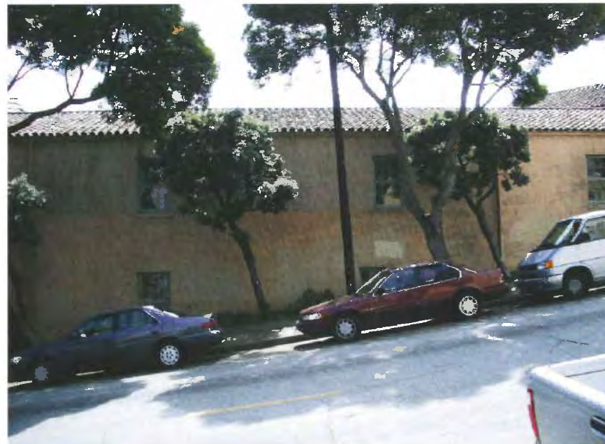
Facade along Haight Street
