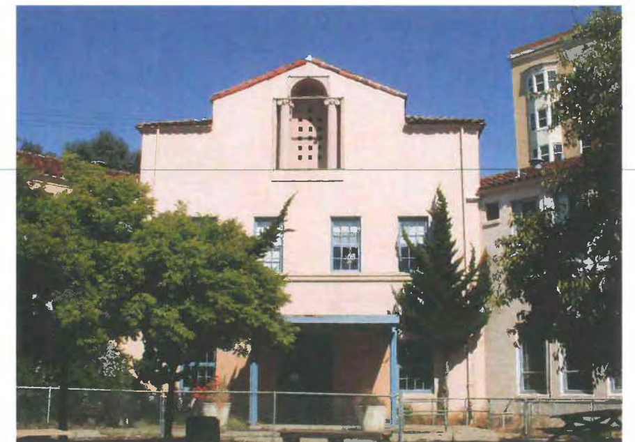
Ionic columns and arch above courtyard entry
