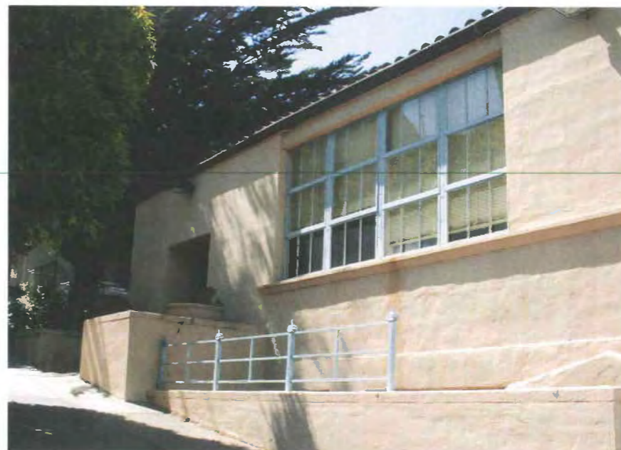
Decorative gate along Hermann Street
