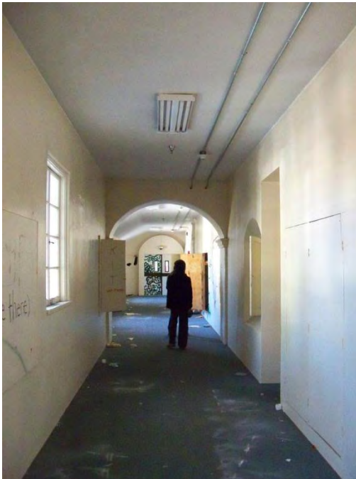
Figure 24. Second floor corridor in Woods Hall Annex, 2012 Source: Christopher VerPlanck
