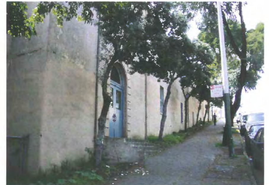
Facade along Buchanan Street
