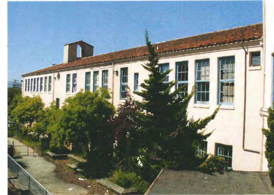
Courtyard facade showing terra cotta roof and wood windows
