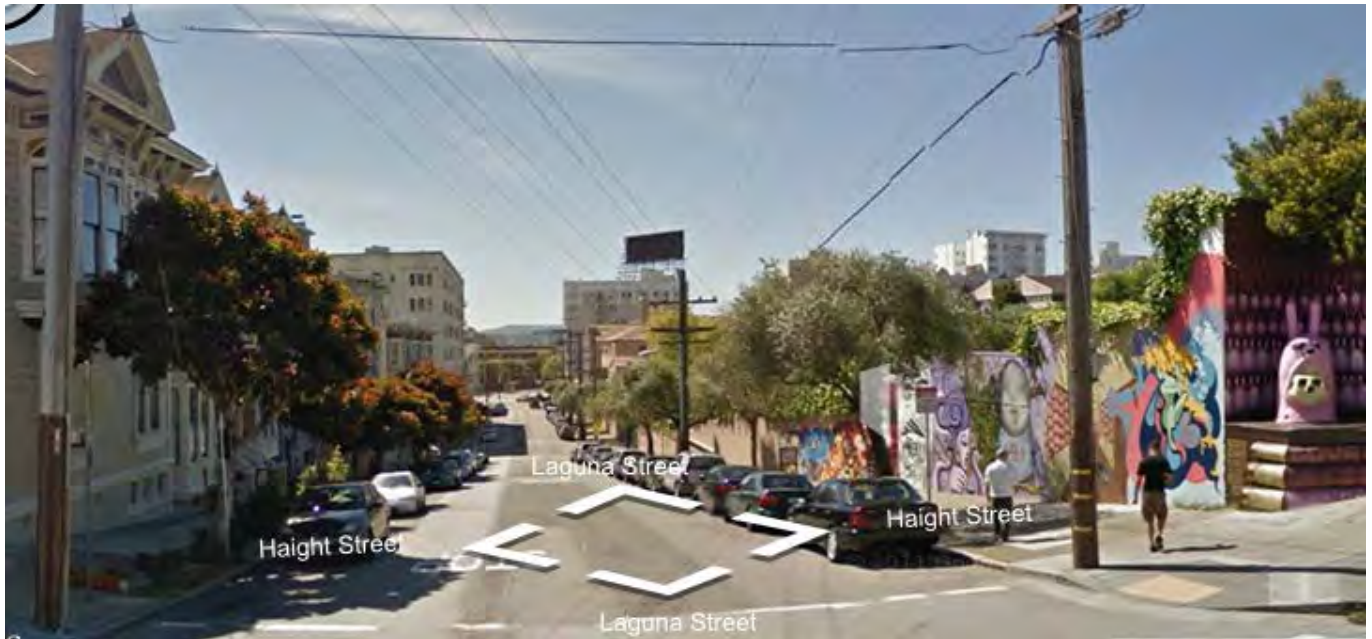
Looking south on Laguna Street from the intersection of Haight Street. Retaining wall to be demolished is on the right.
