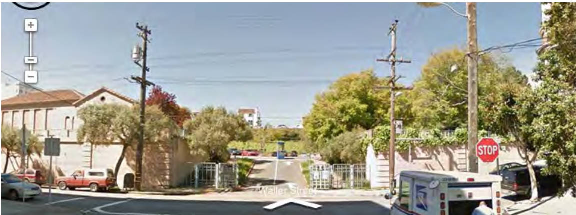
Looking east at the top of the proposed Waller Park. Middle Hall to be demolished is on the left.
