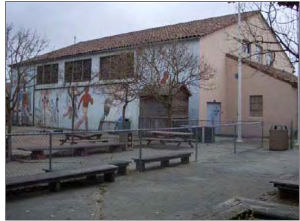
Figure 20B Middle Hall, North Facade
