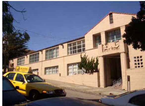
Figure 24B Richardson Hall, South Wing
