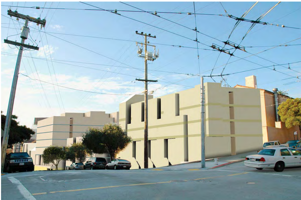
B. Simulated view of the project site from the Laguna/Haight Street intersection looking southwest.
