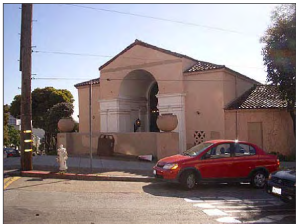
Figure 22A Woods Hall Entry Pavillion at Buchanan and Haight Streets
