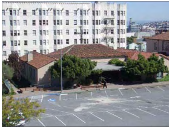
Figure 21 Richardson Hall Administration Wing
