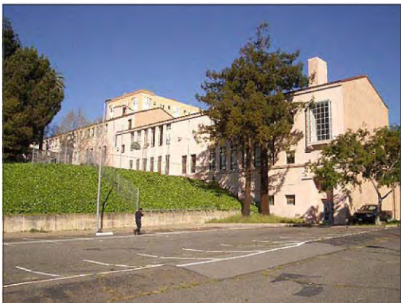
Figure 25A Woods Hall Annex, South Facade
