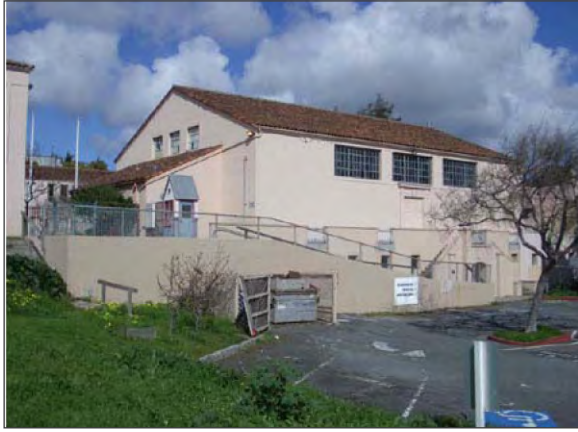
Figure 20A Middle Hall, South Facade
