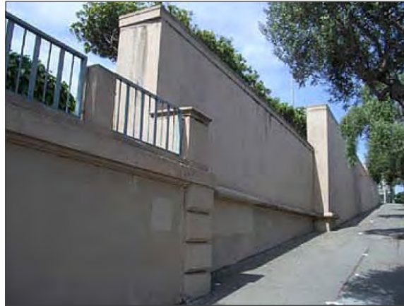
Figure 23 Retaining Wall Facing Laguna Street
