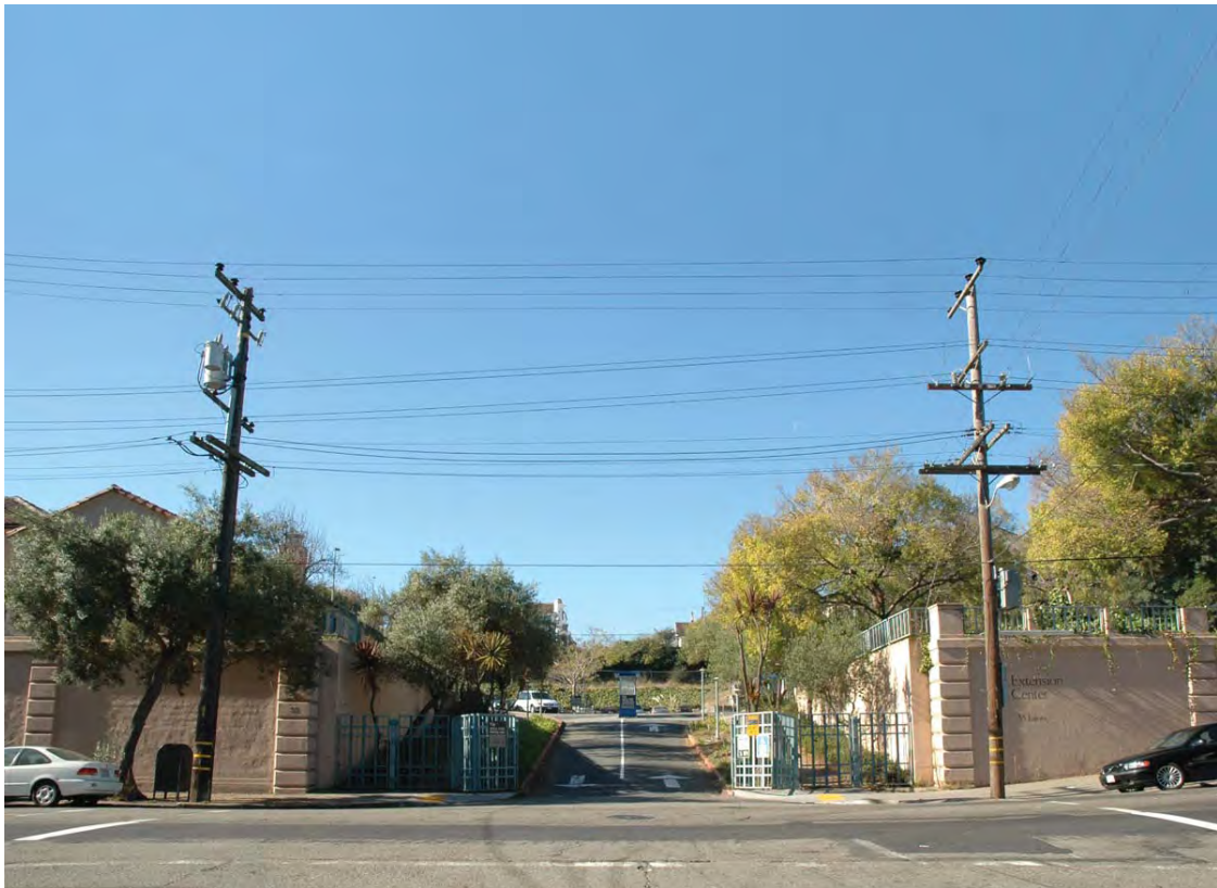
A. Existing view of the project site from the Waller/Laguna Street intersection looking west.
