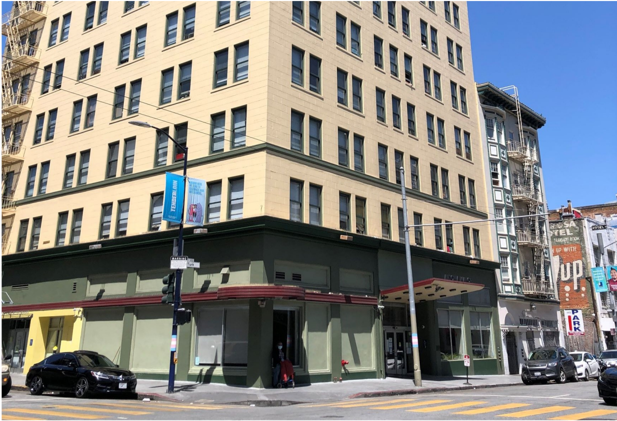
Photo 3 – View of the 10-story Antonia Manor hotel across Turk Street, looking to the northeast.
