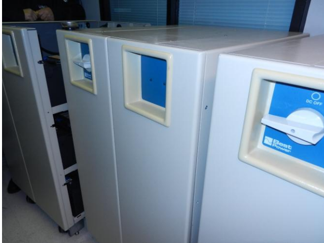
7. UPS Battery Units within SFPCU Building Server Room
