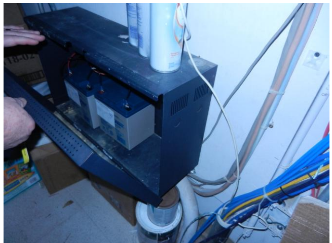
12. Batteries in Fire Alarm System in SFPCU Janitorial Closet
