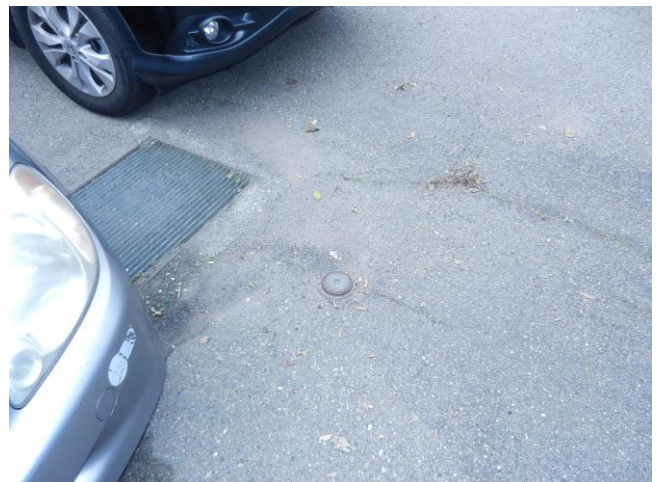
18. Storm Drain with Presumed Adjoining Cleanout on Parking Lot Parcels
