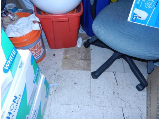
13. Damaged Floor Tile in SFPCU Janitorial Closet
