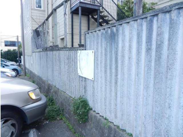
19. Potentially ACM-Containing Perimeter Fencing on Parking Lot Parcels
