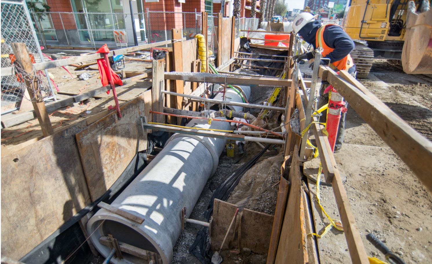
Photo 7.7 New installation of concrete sewer pipes. Robert J. Pierce, SFMTA
