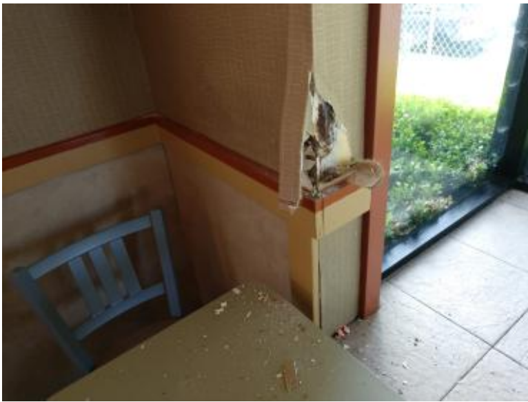
Photo 7 Caption: Tan Wall Covering, Perimeter Greenboard
