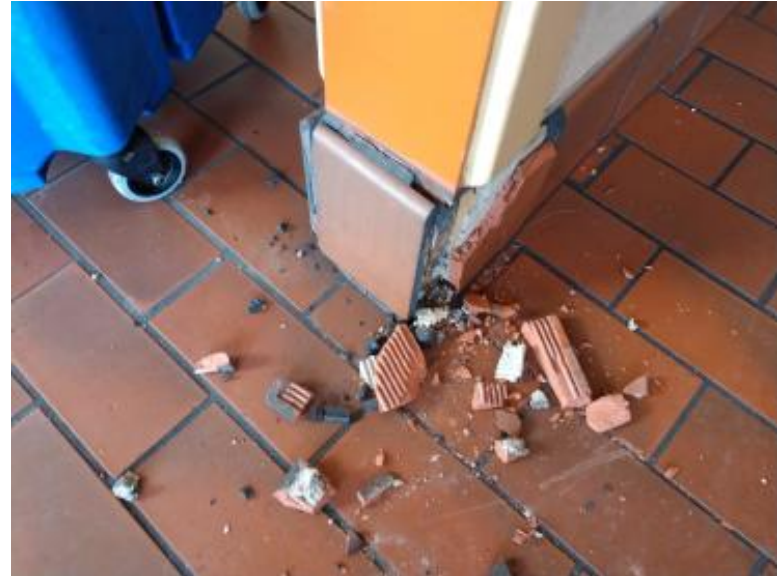
Photo 10 Caption: HMs 5/6 - Ceramic Tile Cove and Flooring Systems
