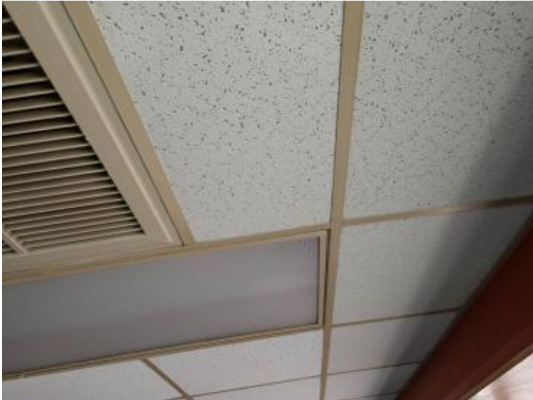
Photo 9 Caption: HM 3 - Lay-in Ceiling Tile System
