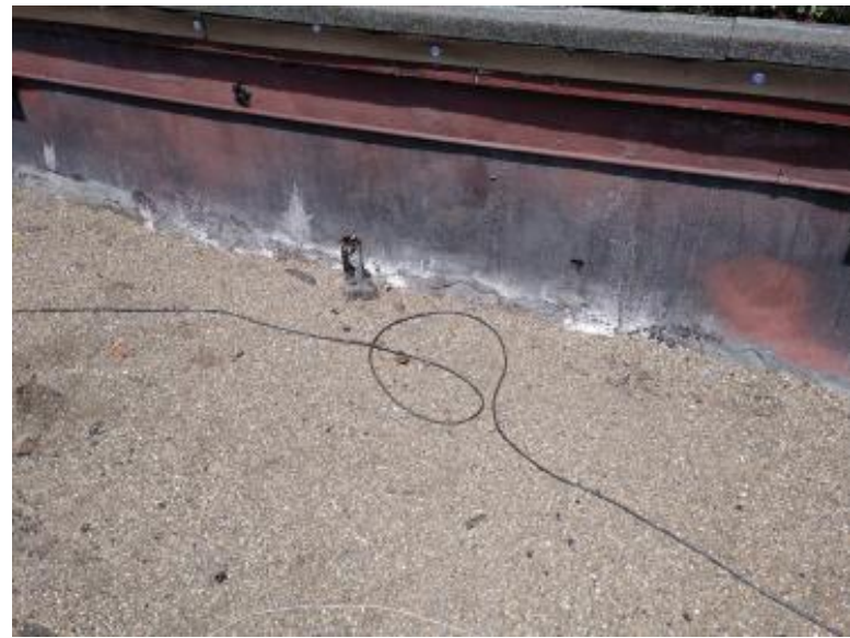
Photo 4 Caption: Main Roofing Field with ACM Roof Mastics
