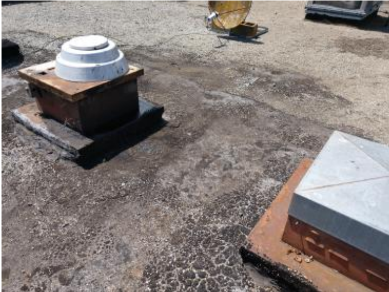
Photo 5 Caption: ACM Roofing Mastics on Main Roofing Field
