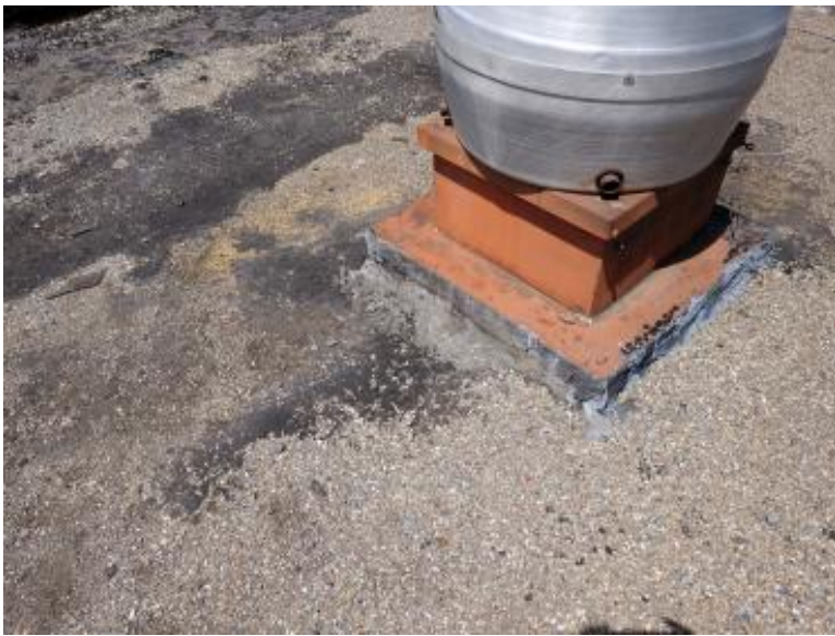
Photo 3 Caption: HMs 31/32 - Roof Curbing with ACM Roof Mastic
