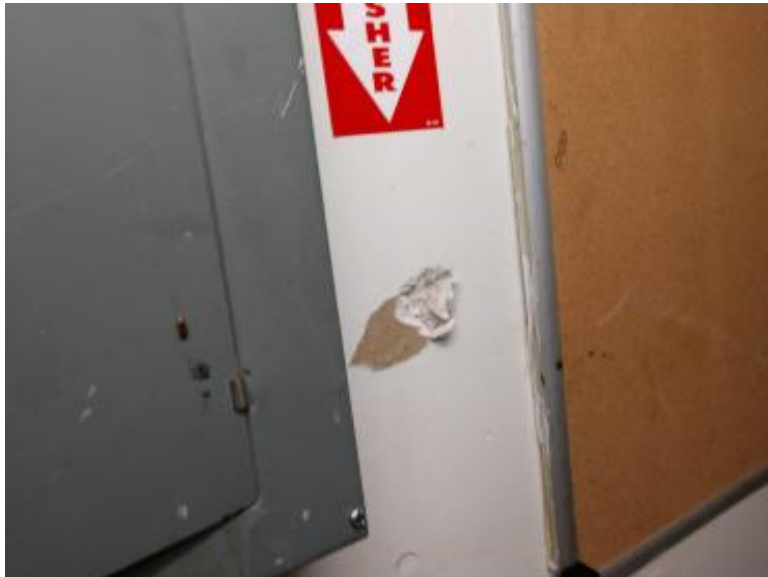
Photo 33 Caption: HM 13 - Drywall Wall System (ACM)
