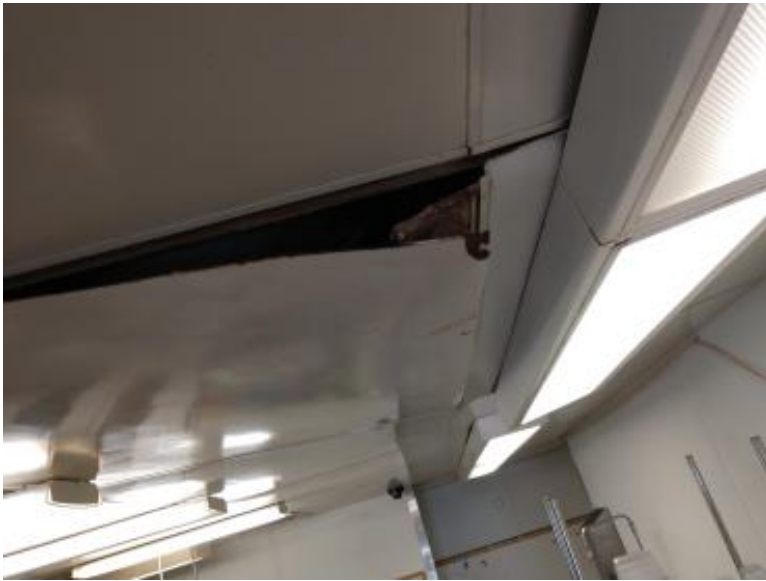
Photo 19 Caption: HM 12 - 4' Glued on Ceiling Tiles
