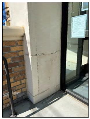
Photograph of some cracking at column of entryway (2-17-22)
