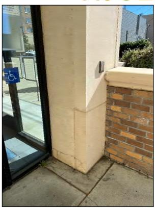
Photograph showing some cracking at column of entryway (2-17-22)
