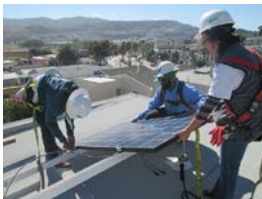
GRID Alternatives installing solar panels
