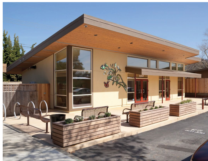
ARBORS APTS COMMUNITY BUILDING
