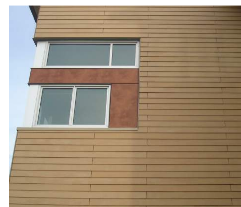
Facade Materials: PNL-1 Slats Installed
