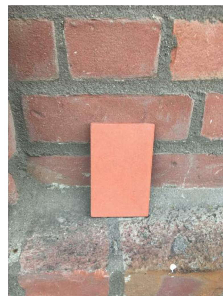
Facade Materials - Brick Context and Panel
