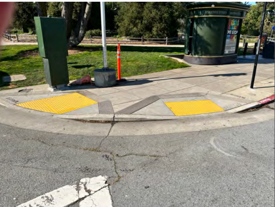
EXISTING CURB RAMPS PHOTOS
