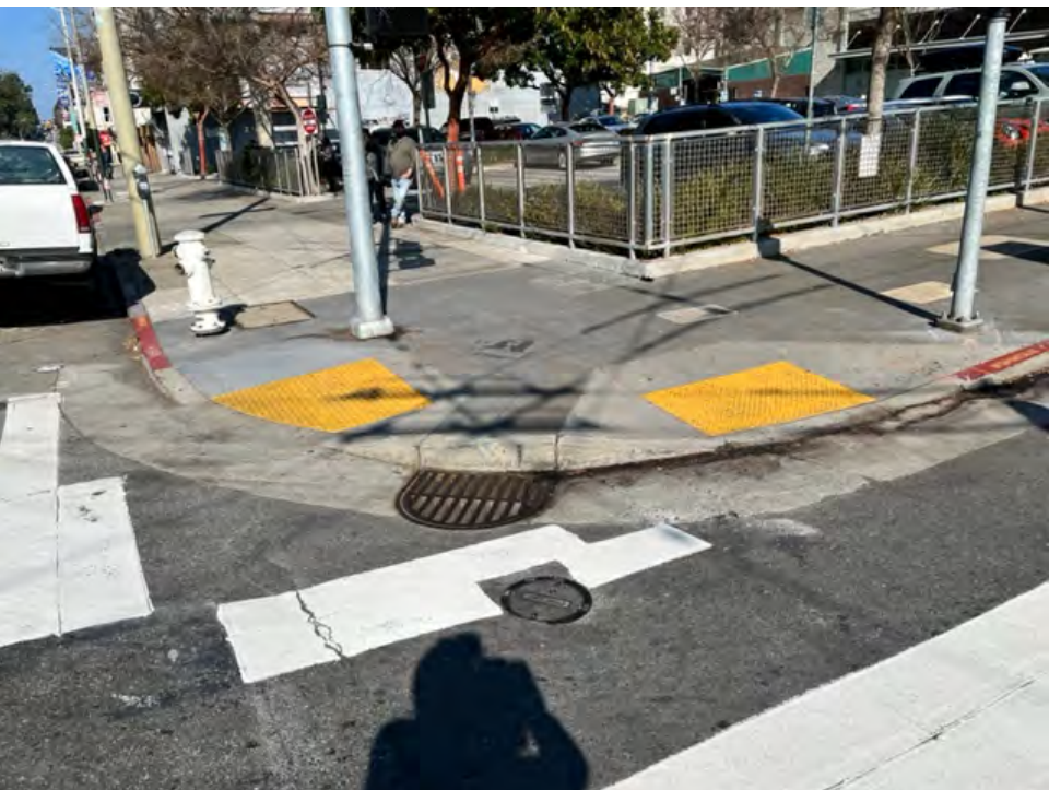
EXISTING CURB RAMPS PHOTOS
