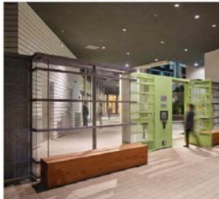
FENCE WITH LOW IRON GLASS INFILL PANELS
