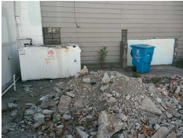
Photograph 5. View of the empty used oil tank located near the northwest corner of the building.
