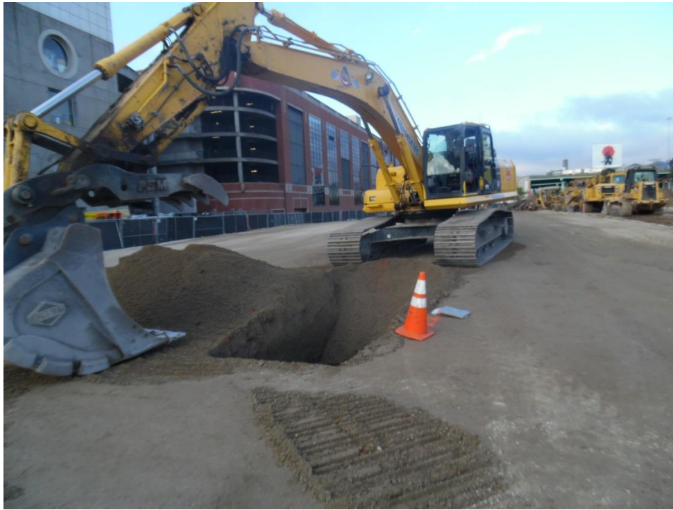
Photograph 7: 5/22/15 - Facing southeast. Excavated test pit for the collection of confirmation soil sample CS-2-05-22-15.
