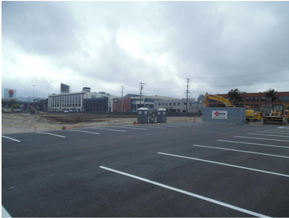
Photograph 5: 5/18/15 – Facing west showing completed asphalt parking lot, crushed concrete partially laid down for the part of the MOH parcel and the earthquake fill further northwest.
