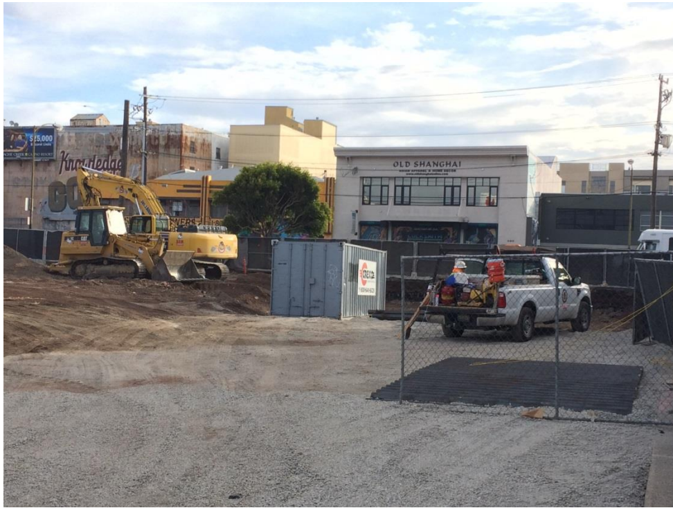
Photograph 3: 5/13/15 – Facing northeast. Gravel is placed prior to asphalt paving.
