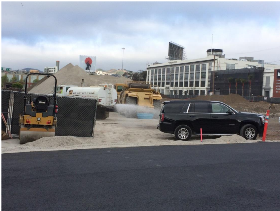
Photograph 4: 5/15/15 – Facing west showing different colors of the asphalt parking lot (foreground), crushed concrete layer (west) and earthquake fill (northwest).
