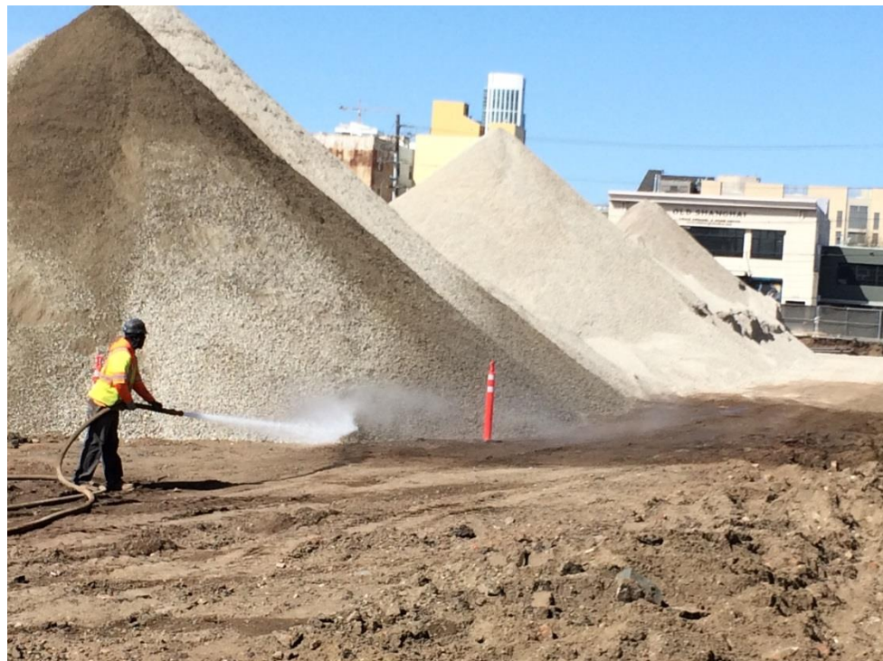
Photograph 2: 5/12/15 – Facing north. Close-up of crushed concrete piles that was used as cap material.
