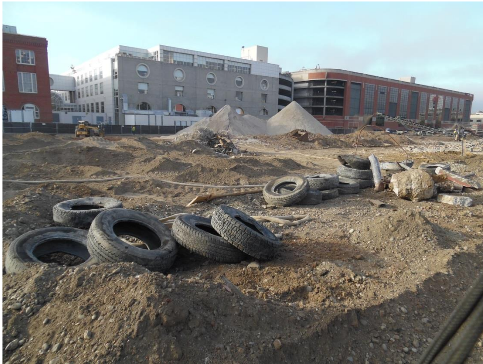
Photograph 1: 5/11/15 – Facing south. Concrete crusher operated by Ferma Corporation Crushed concrete piles that was used as the temporary cap material. Concrete piles are light grey in color compared to the brown earthquake fill.
