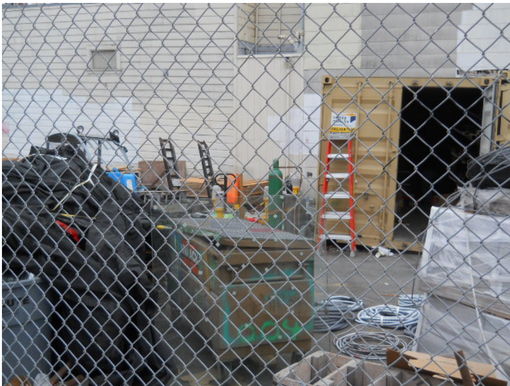
Construction material as seen for the Octavia Street sidewalk.
