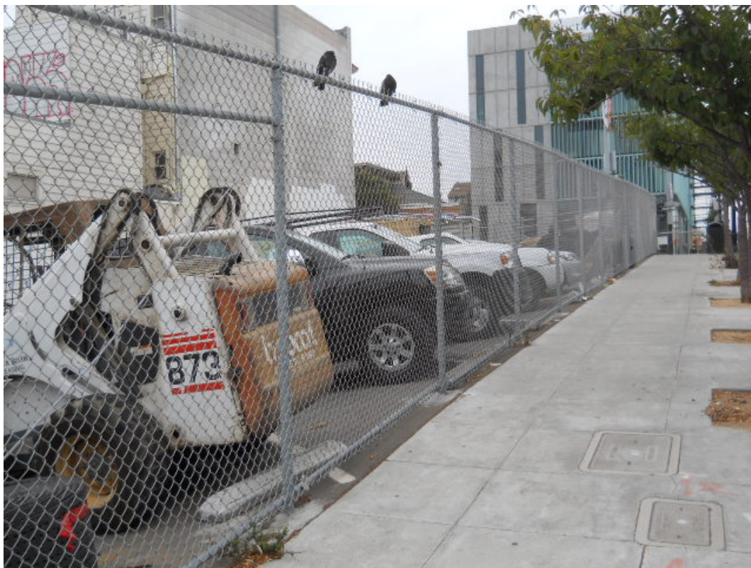
Overview of the west side of the site along Octavia Street sidewalk.
