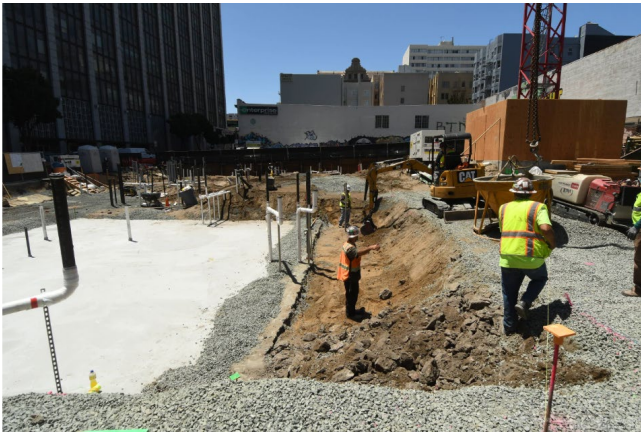
Construction underway at 500 Turk
