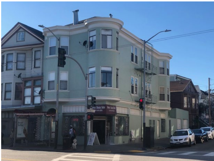
3800 Mission Street – completed June 2019
