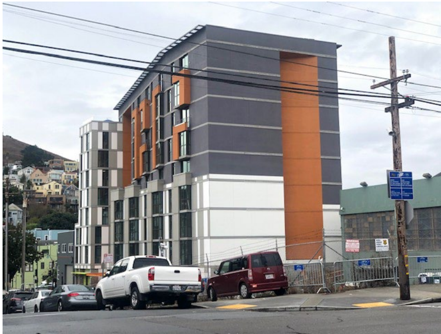
Casa Adelante - 1296 Shotwell construction complete and fully-occupied
